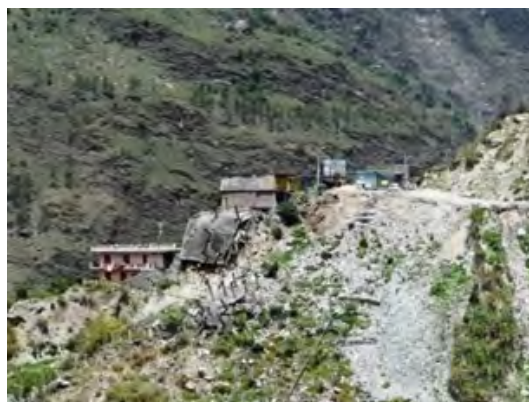
Photo: Houses located on the loose slide material are collapsing
