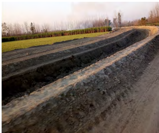
Maintenance of sub-canal in Saharanpur district
