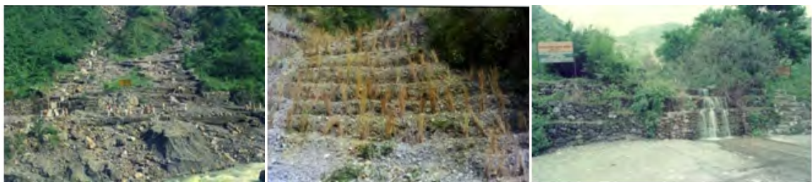
Mine spoil rehabilitation interventions at Sahashtadhara, Dehradun
