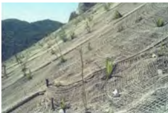
Geojute for landslide control at Sainji
