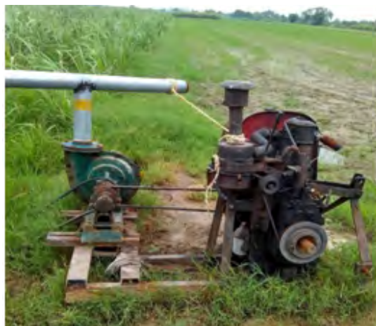
Ground water extraction using diesel engine
