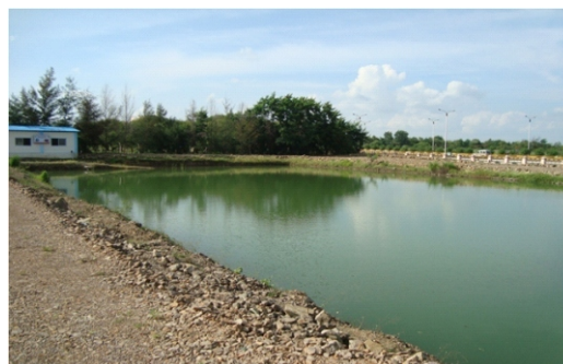
Photo 3. Water Harvesting Structure excavated at ICAR-NRCP, Solapur
