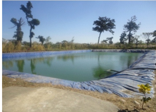
Submersible Pump in Floating Platform
