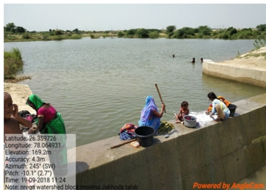
Photo 1. Collection of rainwater in pond constructed under NREGA scheme
