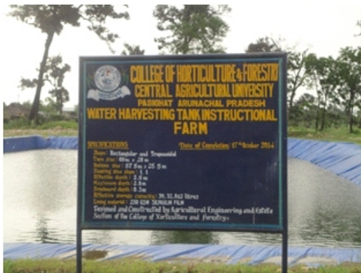
Harvesting of in-situ rainwater in the water harvesting pond
