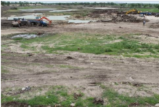
Silt being removed from the bed of the tank in Vanaparthy GP
