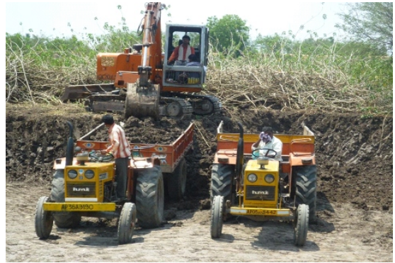
Silt being removed from the bed of the tank in Vanaparthy GP
