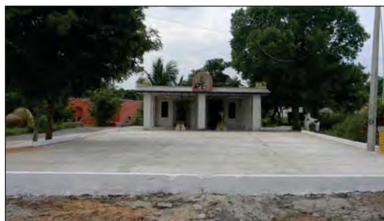
Work : Construction of Thrashing Floor Village : Mallagunda ; Amount ₹ : 1,50,000/-
