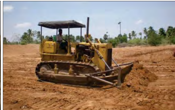
Bulldozer for Land Development
