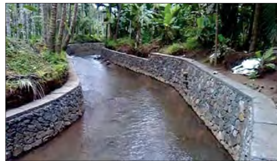
Retaining wall in Pazhayanooppadam Thodu
