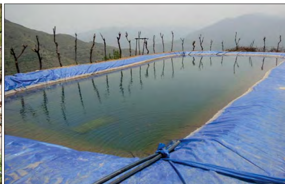
Water Resource Development in Sainj Village
